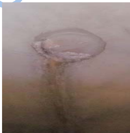
Leak stain on water tank
