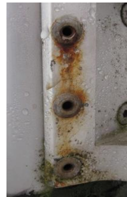
Vang rivets corrosion stains
