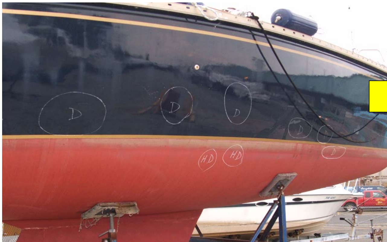
Chalk circles show areas of concern on the starboard side. “D” = dull checking. “H” = extremely high moisture levels.
