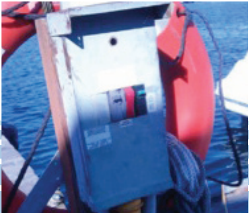
Circuit breaker should not be taped in the on position. This eliminates the safety feature of the product.
