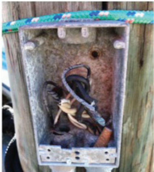
Exposed cables or electrical boxes should be closed.
