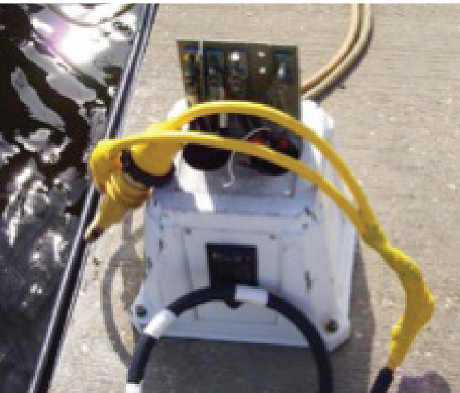
Exposed electrical connections can lead to a potential safety hazard.
