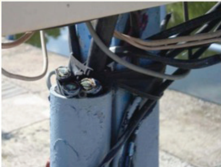
If electricity is turned on, exposed conductors can be potential safety hazards.
