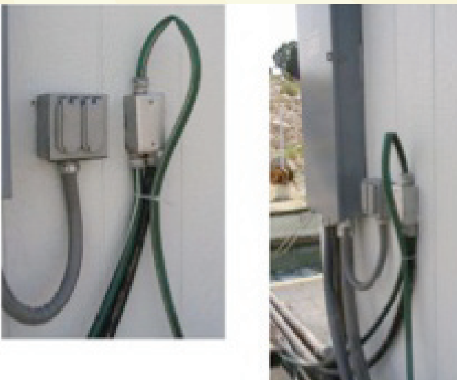
Exposed electrical connections can lead to a potential safety hazard.
